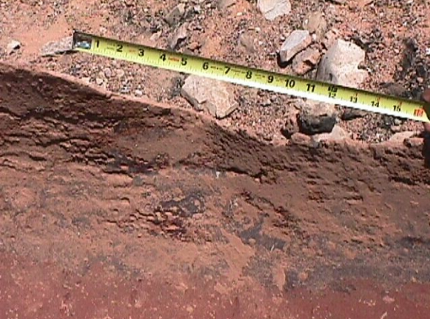
Photo #3 - inside of pipe
