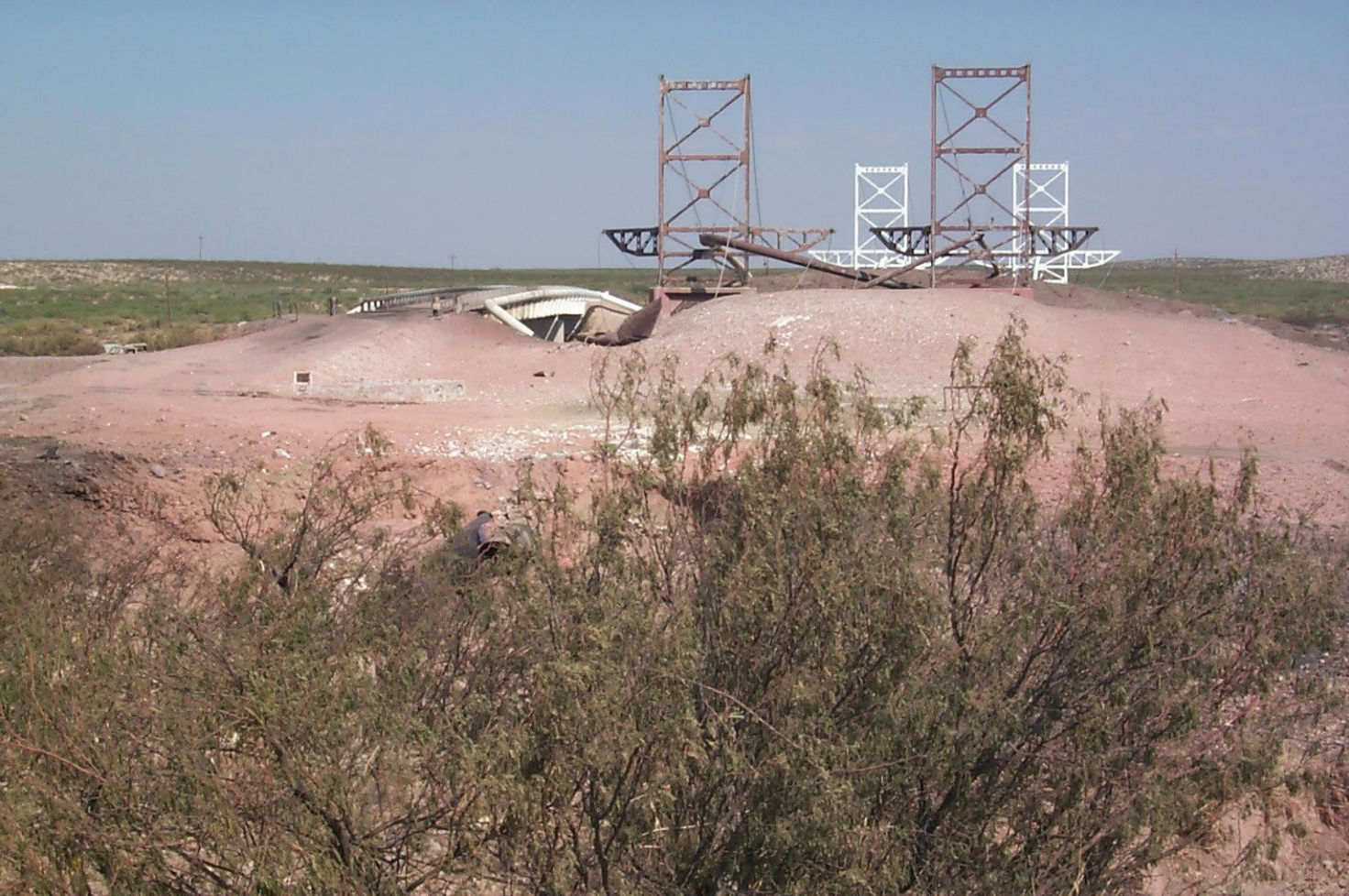
Photo #5 - concrete bridge and pipeline suspension bridges, taken from east side of Pecos River
