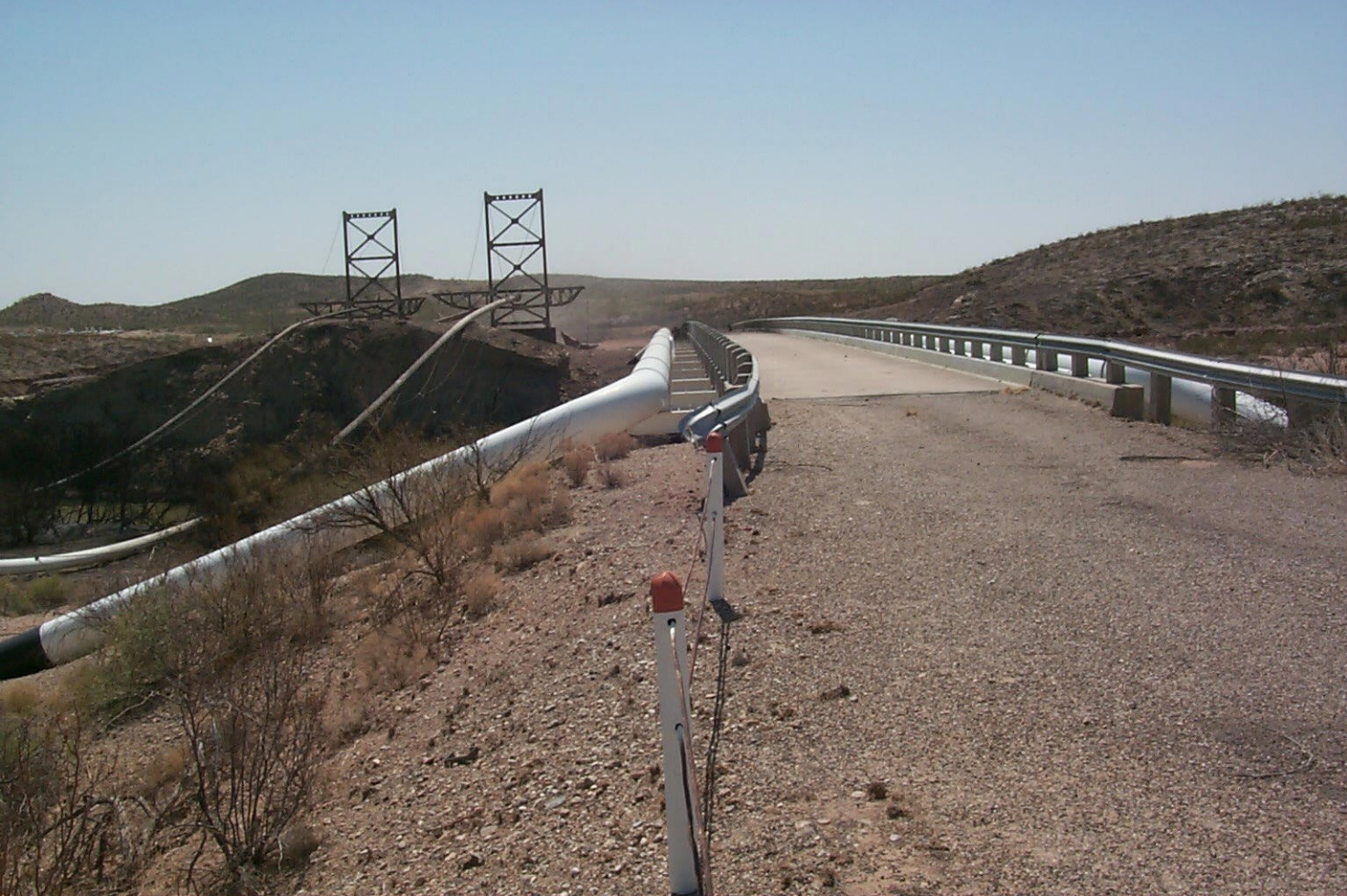
Photo #6 - line 1103, concrete bridge and pipeline suspension bridges, taken from west side of Pecos River
